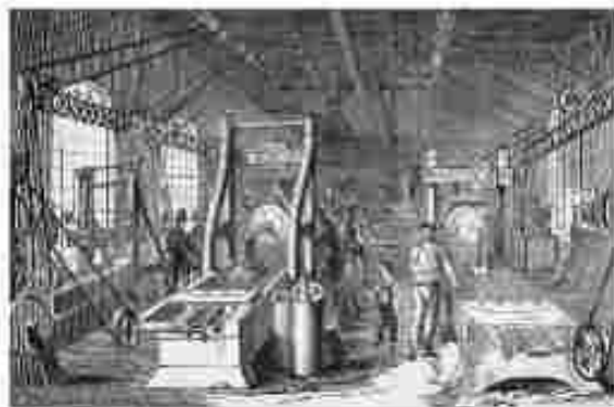
Fig. 6 - A fitting shop at a railway works in England, The Illustrated London News, 1849. In the fitting shop new locomotive engines were completed and old ones repaired.
